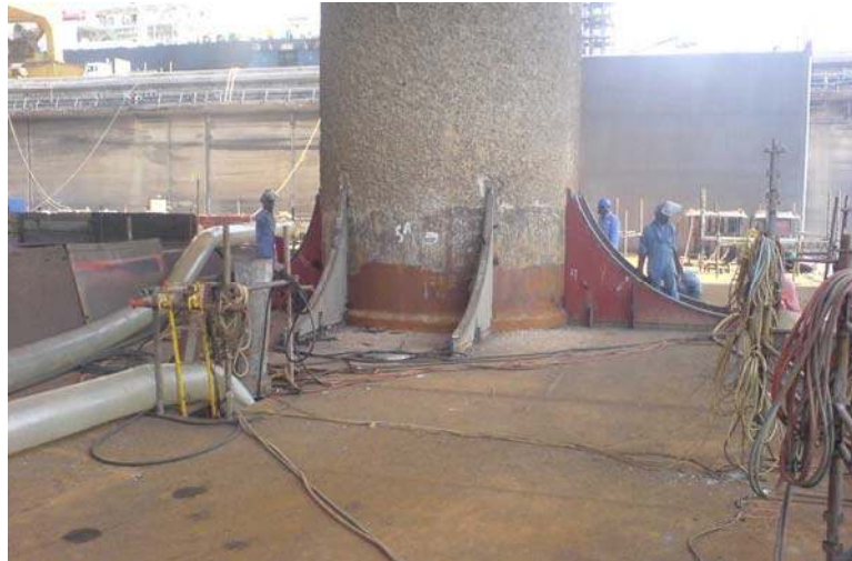
Figure 3: Retrofitted Mat-Leg Connection (At Top of Mat)
